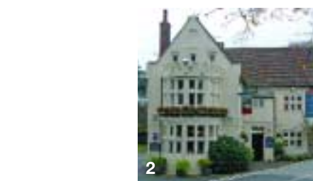
1 The Old Vicarage: stone Venetian window over stone pediment of doorcase 2 Woolpack Inn 3 White Horse Inn
