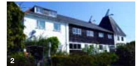
1 Whittington and Rosecroft cottages 2 Dwellings in converted oast houses 3 Stowe Cottage 4 North Court Fruit Farm
